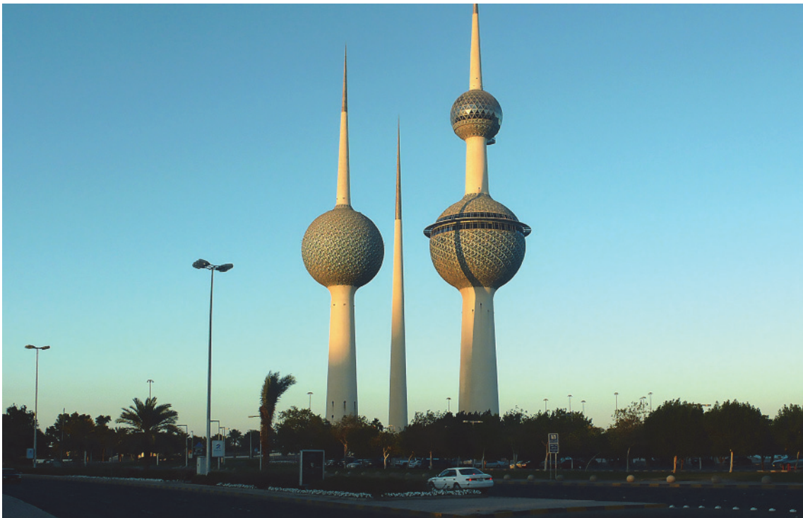
Kuwait villa, 1960s (Photo: © Ghazi Sultan) and Kuwait Towers, 2007.
